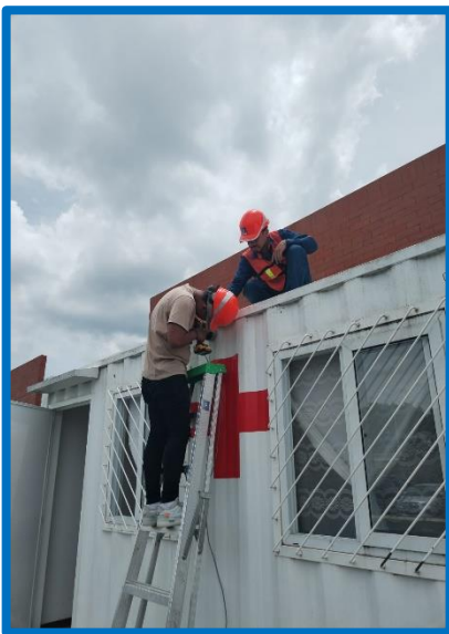
Hospital de Chimaltenango
